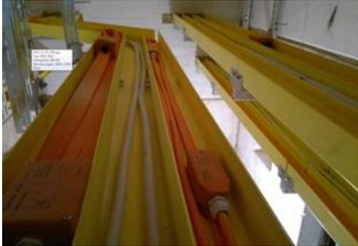
For London underground the requirement for circuit integrity was EN50200 and BS8434-2 but not DIN4102.
